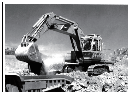
photo 2.1 — A hydraulic excavator in operation in a rocky-soil ground
